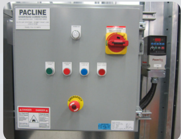
PACLINE control panel with the VFD mounted externally to allow the flexibility to adjust the conveyor speed quickly.
